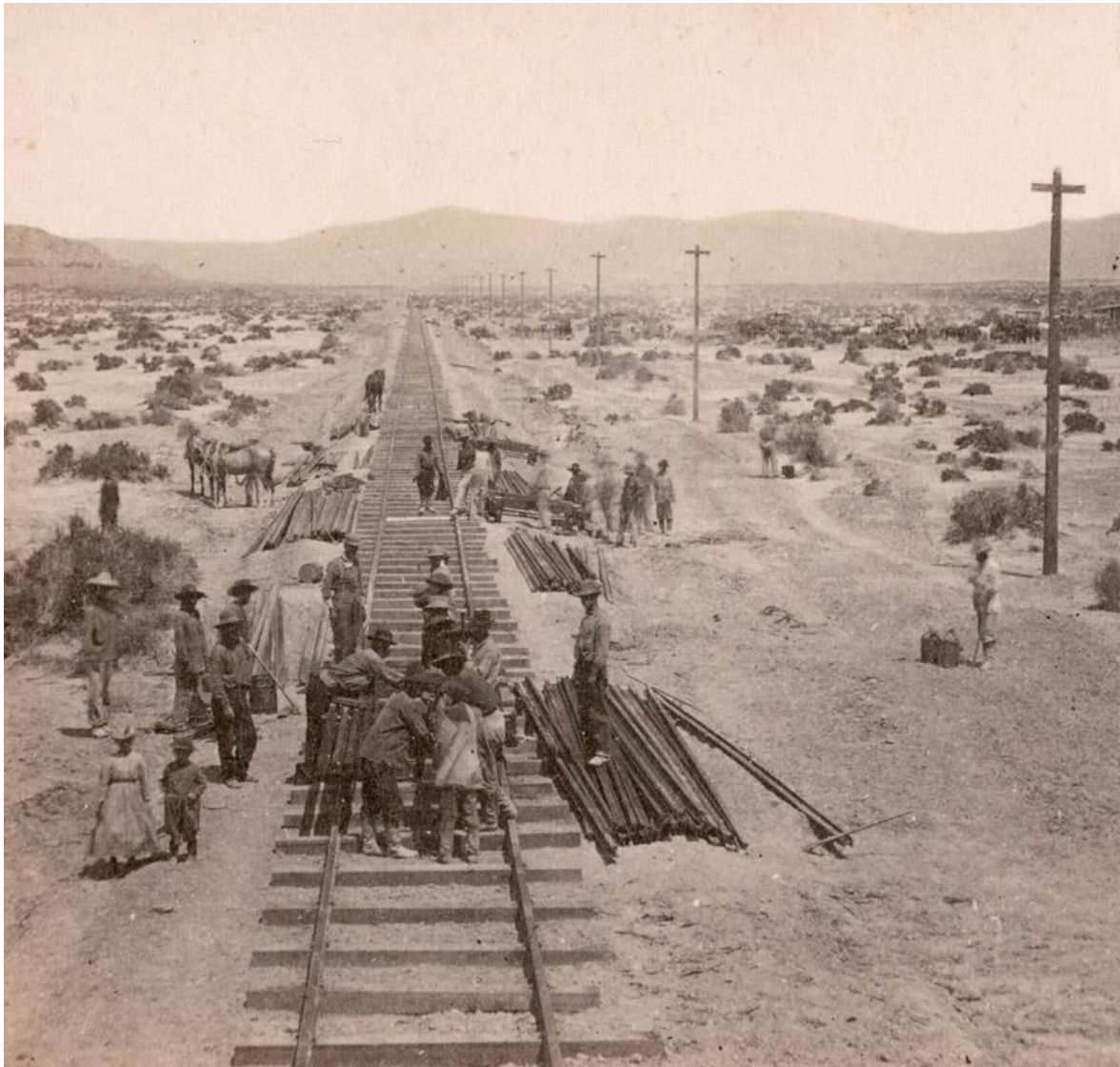
Construction of the transcontinental railroad helped establish the precedent that the government would provide as much assistance as necessary to allow private investors to finance the line. In this photograph, workers for the Central Pacific Railroad lay track near Humboldt Lake in northwestern Nevada. (Courtesy of the California History Room, California State Library, Sacramento, California.)
